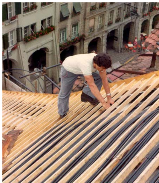
Figure 7-4 Roof collector below tiles installed between rafters, 1978 [Grimm 2007]
