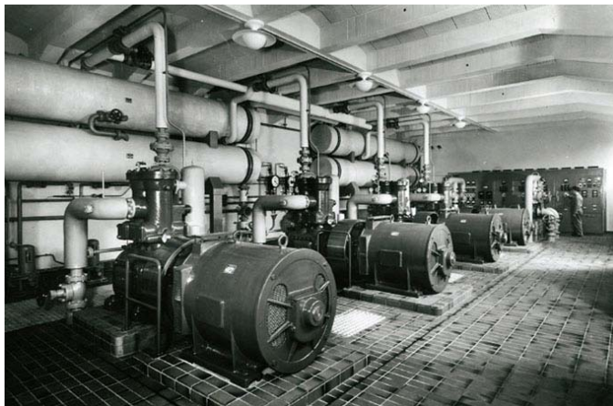
Figure 5-22 Machine hall with heat pumps and condensers, 1943 [Eberhard 2007]
