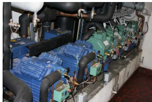
Figure 8-22: Compressors of the investigated plant example [KWT, CH-3123 Belp]
