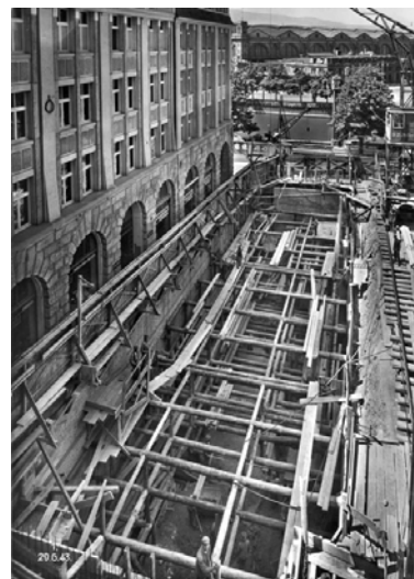
Figure 5-18 Underground machine room under construction, 1942 [Riesen 2007]
