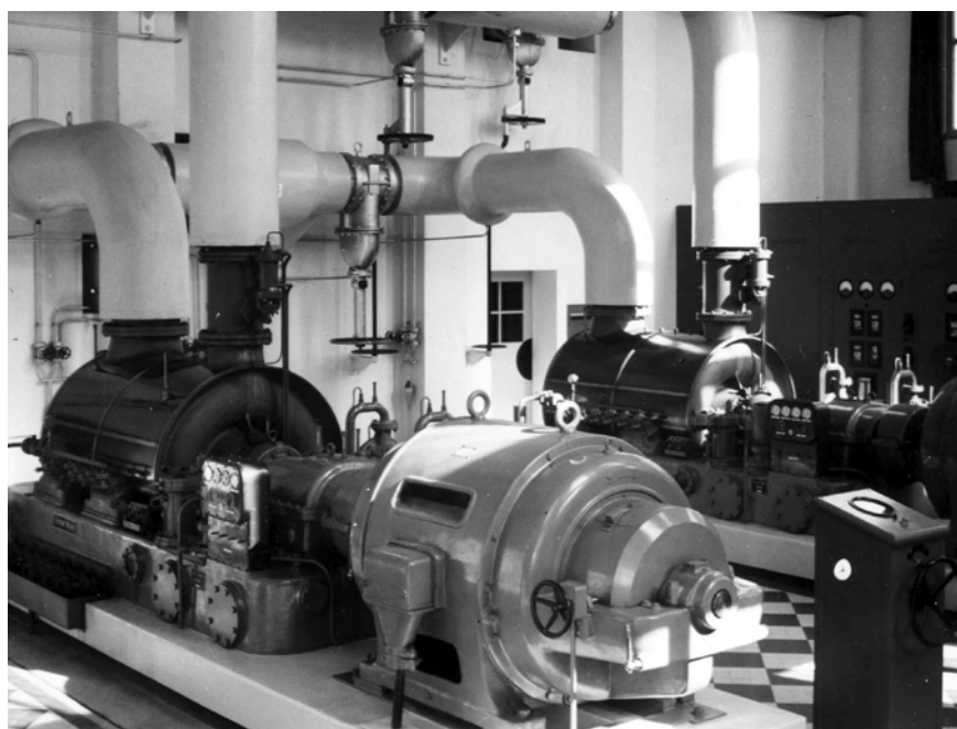
Figure 5-24 Compressor station, Swiss Saline Riburg, 1941 [Lieberherr 2007]
