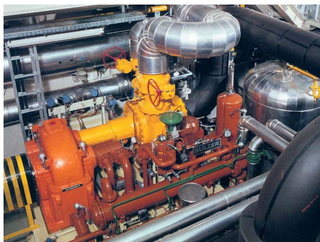
Figure 5-16 Heat pump unit since 1988 [Friothers 2008]
