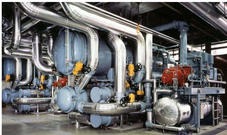
Figure 7-13 3.9 MW ammonia heat pumps at EPFL, 1986 [Friothersm 2008]
