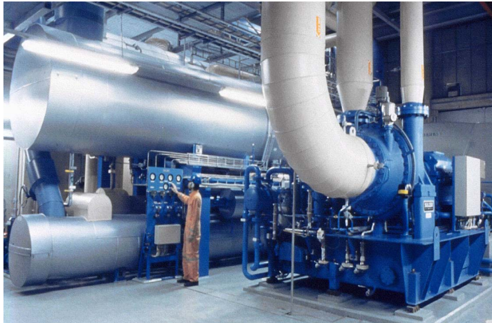
Figure 7-14 One of the six 30 MW radial compressor heat pump units of the Värtan Ropsten district heating system of Stockholm [Frio-therm 2008]
