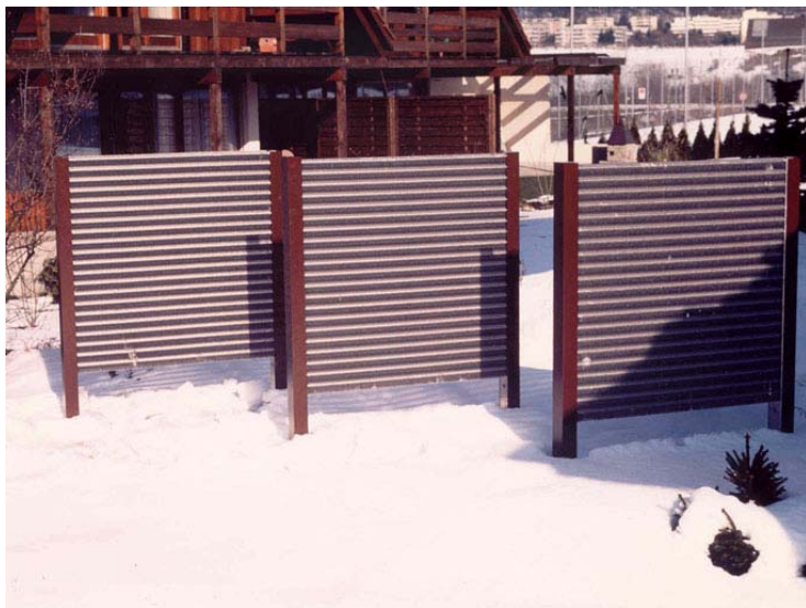
Figure 7-6 Energy fence evaporator type around 1980, Neucalora [Grimm 2007]
