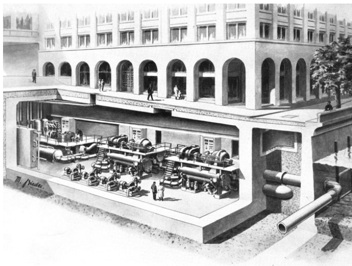
Figure 5-17 5.86 MW heat pump plant at Walche, 1942 [AFB 1988]
